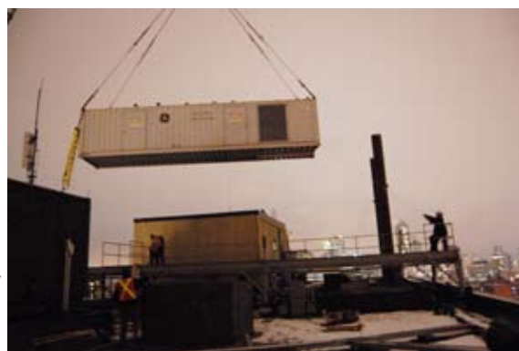
Combined heat and power unit is lifted onto the roof of the David A. Croll apartments.
